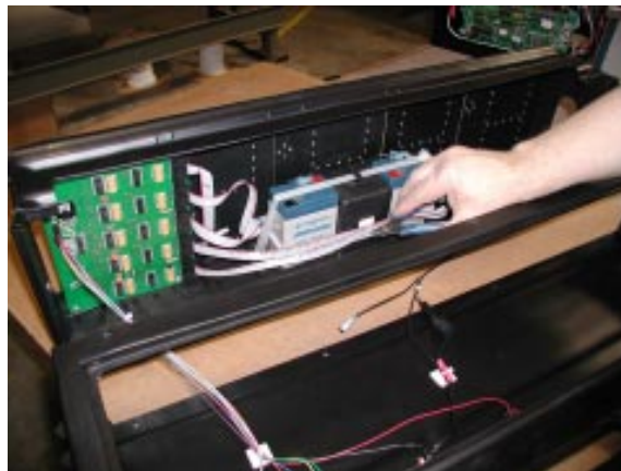
Cut the ribbon cable tie-wrap
