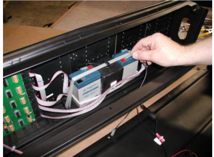
Install the two power wires
