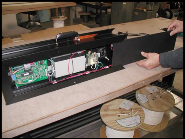
Test the clock and then replace the window and back panel.
